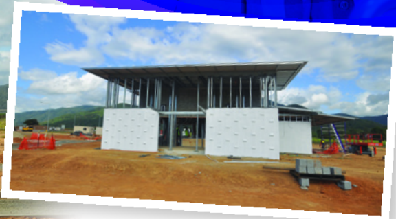
Administration Officer Tina Kalac and Principal Luke Reed inspect the administration block under construction.
